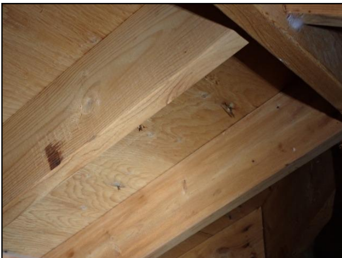
Rafters -Joists - Plywood sheathing
