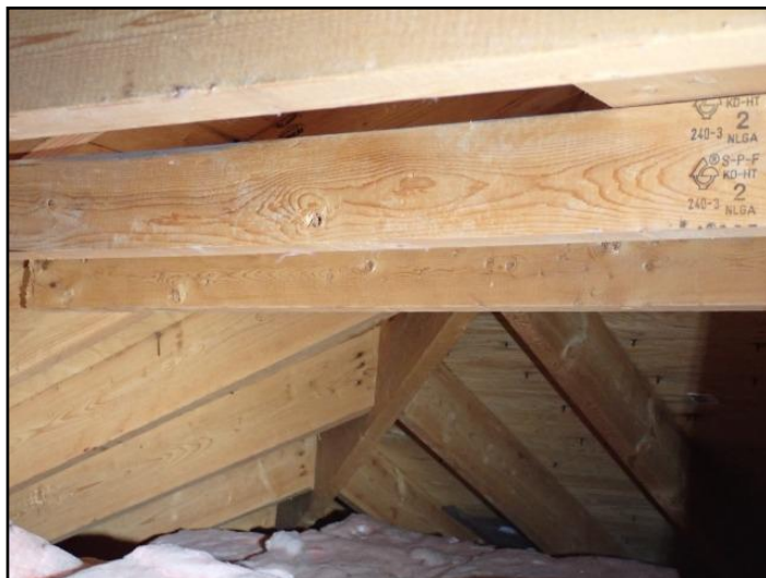
Rafters - Joists - Plywood sheathing
